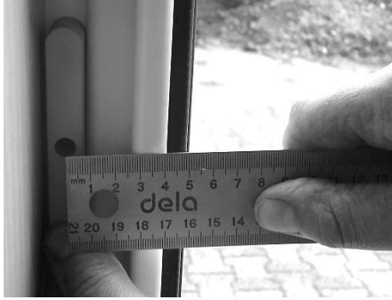
1 – Measure Dimension A (in this case, 50 mm)
