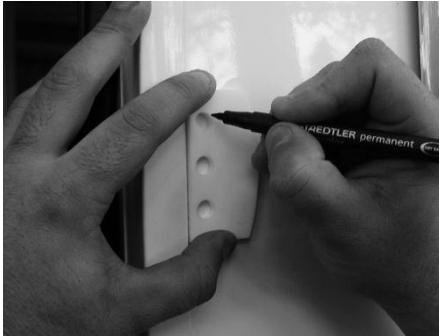
5 – Mark and drill three holes of Ø 9 mm
