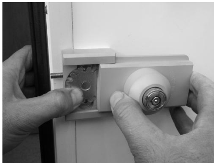
9 – Fit the slide in place by pushing on the Pinion
