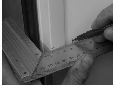
2 – Transfer the resulting Dimension A to the exterior
